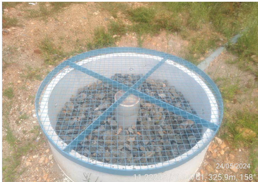
Rain Water Harvesting Units
